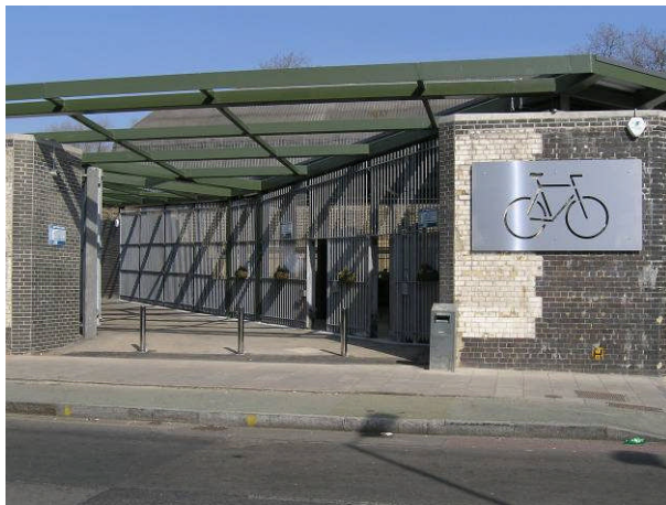
Finsbury Park Cycle Station – access is made secure by the use of smart card control
