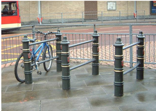
Stands formed from bollards and horizontal bars
