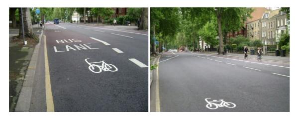
Bus lanes allow cyclists to ride in a safe and assertive national standards position. Putting cycle logos in bus lanes renders the bus lane unenforceable; however a clever way of getting round this and keeping the bus lane legal is simply to place logos at any gaps in the bus lane.
