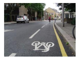
Here the centre lines were removed in order to give room to replace the narrow kerbhugging cycle lanes with wide ones.
