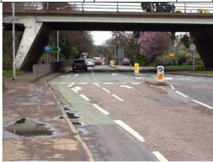
Cycle lanes should not be discontinued on the approach to junctions, better to maintain the cycle lanes at the expense of traffic lane width (traffic may over-run if needed).
