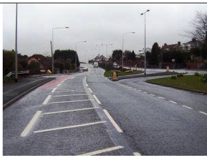
Traffic lane removed from former two-lane configuration to create wide advisory cycle lane with buffer strip.
