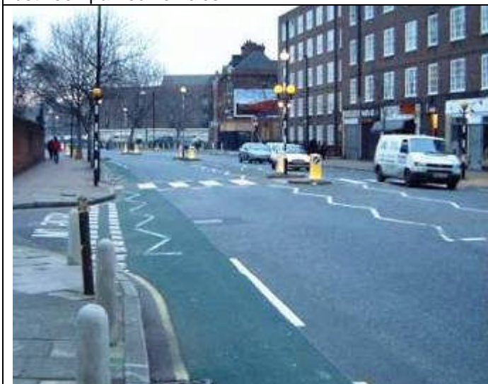
Maintaining cycle lane continuity through crossing zig-zag markings ('virtual cycle lanes') by extending pigment through the markings in place of the cycle lane lines.
