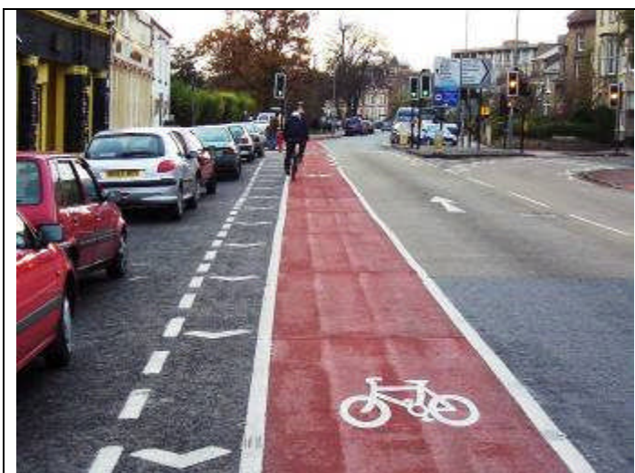
1.5m mandatory cycle lane with additional buffer strip between parked vehicles.
