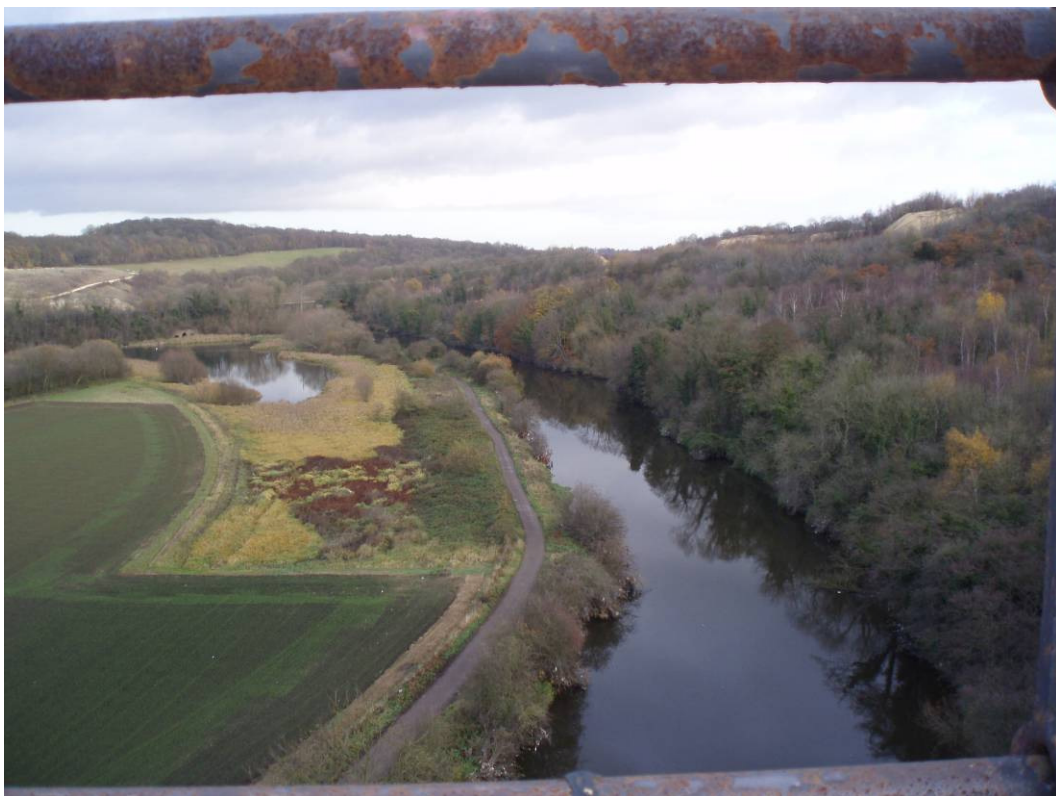
View of the Trans Pennine Trail NCN 62 path along the River Don from the open section of the Conisbrough Viaduct
