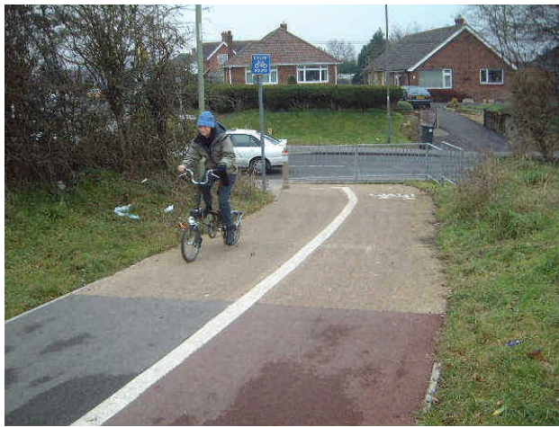
Anti-skid surfacing on approach to road junction, Eastleigh
