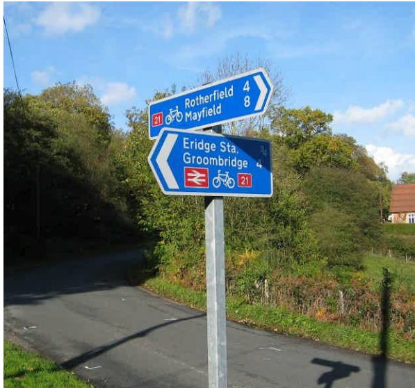
Signs mounted on square posts to prevent rotation, East Sussex
