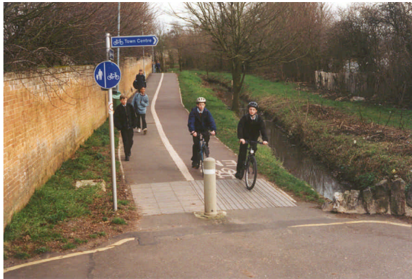
Single bollard to prevent unauthorised car access
