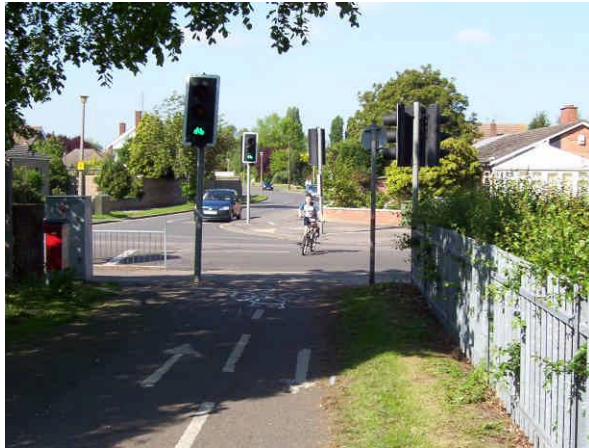
Dedicated light-controlled crossing, Bedford
