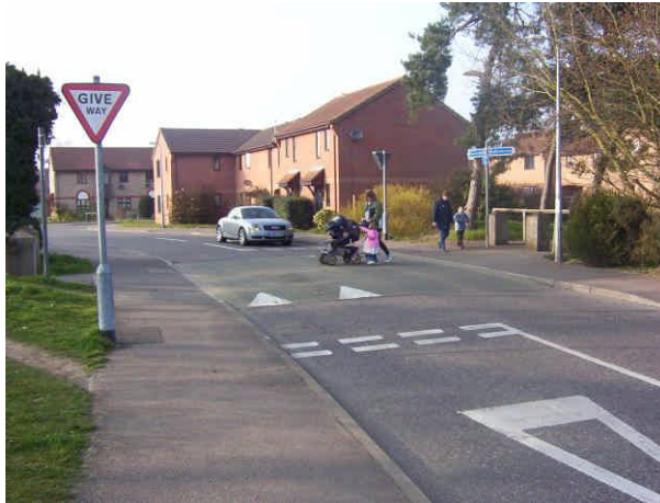
Cyclist priority junction on flat-topped road hump, Thetford
