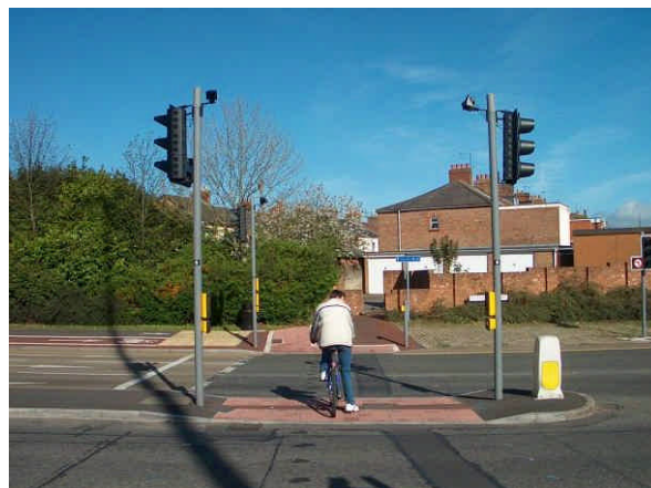
Cycle/pedestrian crossing with central refuge and near side aspects within signal controlled junction, Taunton
