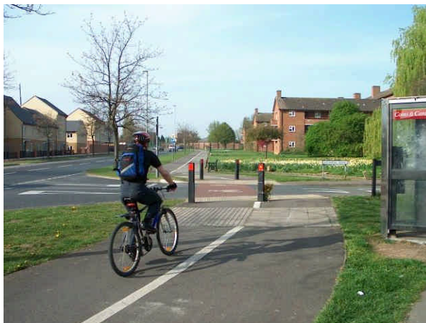
Bent-out cycle track crossing with cyclist priority, Cheltenham
