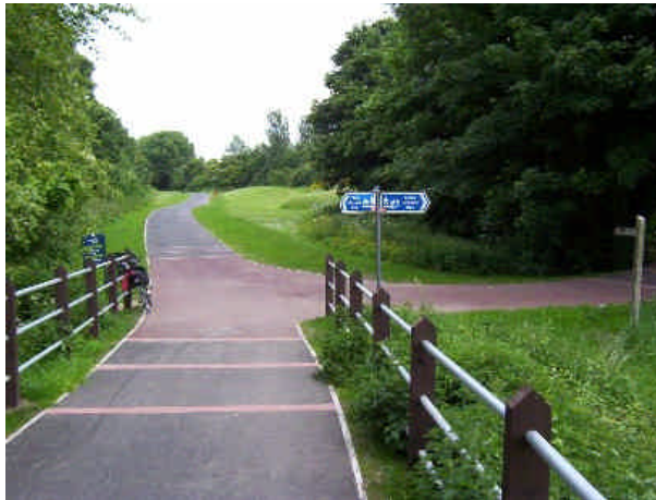
Junction highlighted with coloured paving
