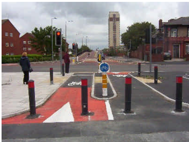
Cycle gap at a signalised junction, Bootle
