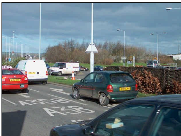
Visibility to the right reduced by means of sight screens, Taunton
