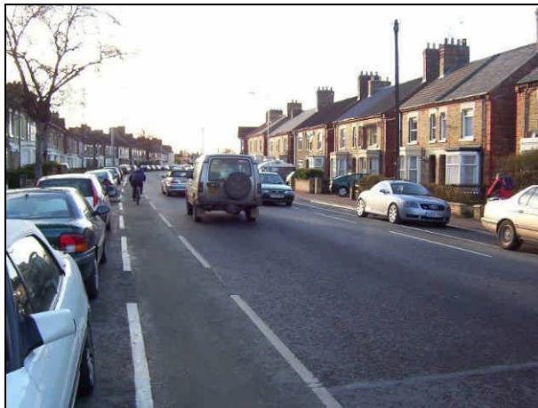
Removal of Road Centre Lines, Peterborough (note absence of buffer zone between parked cars and cycle lane: see A11 Cycle Lanes )
