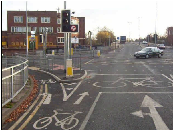
Bypass for cyclists at signal controlled junction, Scunthorpe
