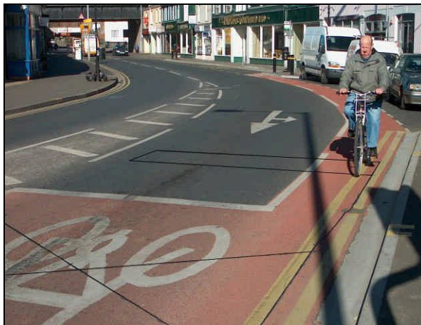
Loops in the road located to detect cyclists, Taunton
