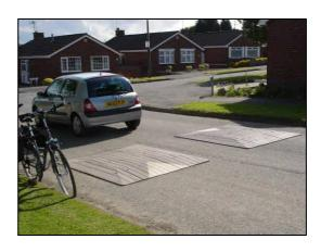
Alternatively, speed cushions could be considered in place of full-width road humps. These are generally more comfortable for cyclists to negotiate than full-width road humps since they can usually avoid riding over the cushions. Usually placed in rows of two or more units across the road, cushions are also sometimes used singly where physical features, such as central traffic islands, limit the usable width to one lane.
