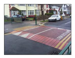
Flat-topped hump using preformed sinusoidal units
