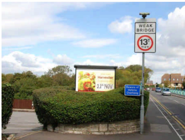
Wide footway at the southern end of the bridge on the western side
