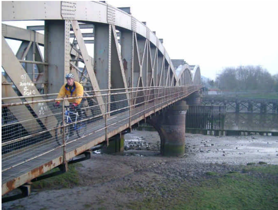
Bridge bolted on to existing structure - Wales
