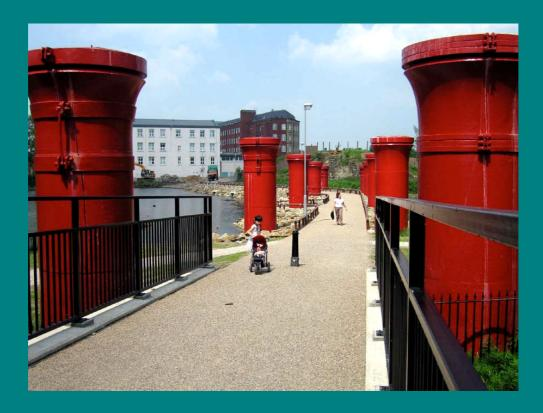
A disused railway viaduct has been remodeled to create a traffic-free route into the centre of Hyndburn. Note the absence of segregation for cyclists and pedestrians, which would have involved additional signage and lining, and the minimalist unauthorised user access controls.
