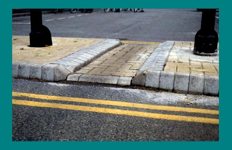
More road closure treatment, although the sharp upstand through the cycle gap is likely to cause discomfort. Although it is unfortunate that it has been deemed necessary to have double yellow lines to keep the way through clear for cyclists.
