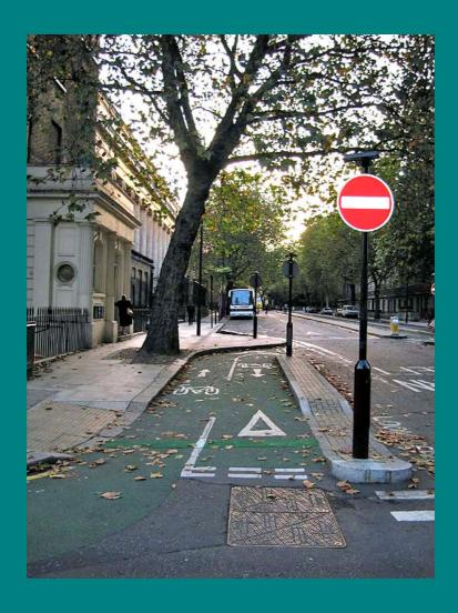
The usual response to enable cyclists to avoid a No Entry sign, in line with DfT regulations (which do not permit an 'Except Cycles' exemption plate on a No Entry sign), is to construct a cycle 'plug', which can be awkward to use and difficult to maintain.
