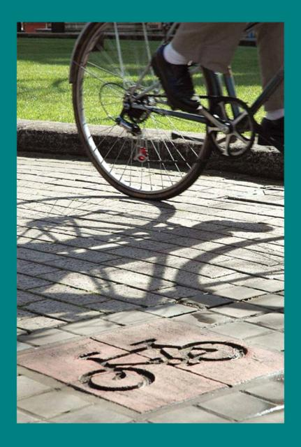
Some of the most durable and vandal-proof 'signage' for cyclists, particularly in urban areas, is embedded in the riding surface. The example here, from College Green in Bristol, has obviously been designed to take account of the wider architectural / aesthetic setting.
