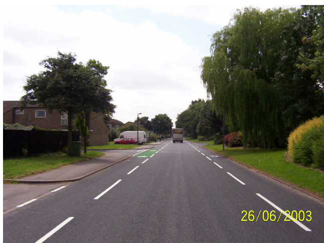
Bristol Road, Scunthorpe: 4.3m two-way central lane bounded by 1.5m wide advisory cycle lanes
