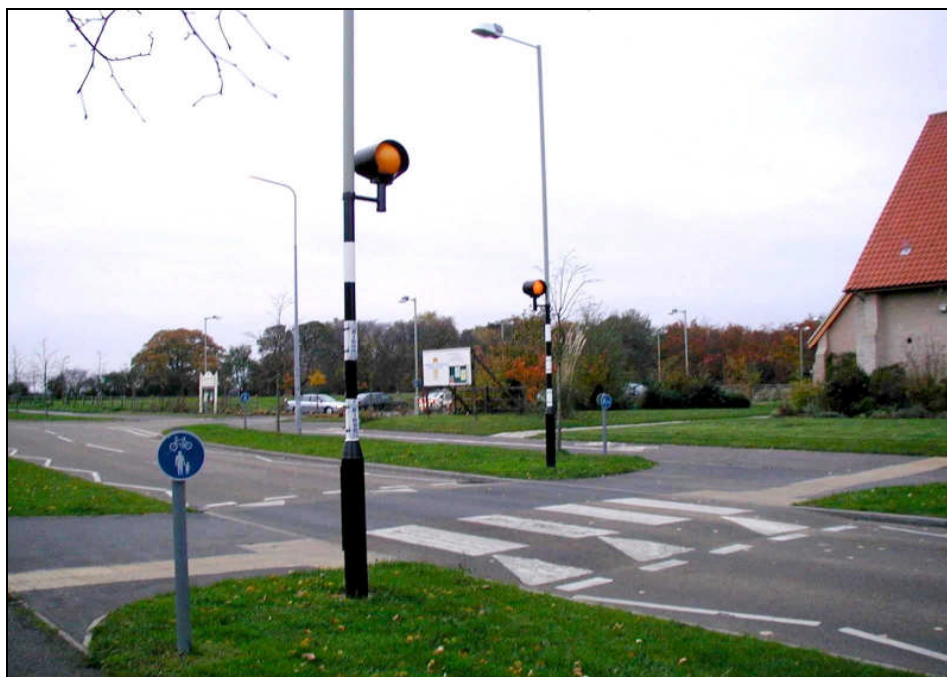
One attempt to create a 'cycle zebra'. Note that this design does not comply with current crossing guidelines.
