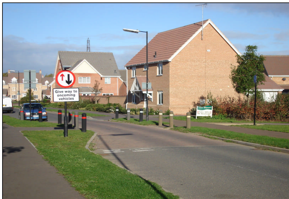
Example of a ramped, give-way crossing (with priority working for traffic) on a new residential development in Peterborough. Photo: Rob Marshall.
