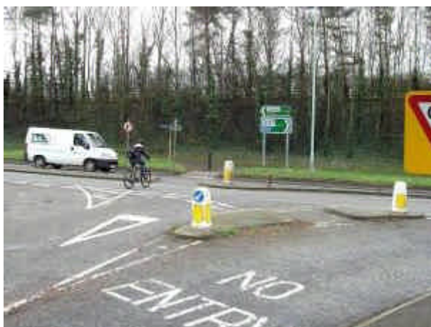
Junction of A358 and Ruishton Lane viewed from the north western side of the junction showing cycle track within the southern verge
