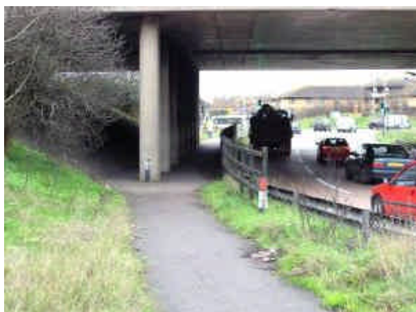
Existing cycle track on outer, south western side of roundabout – cyclists and pedestrians can pass either side of pillars (1.1m wide to left of pillars and 1.7 wide next to carriageway)
