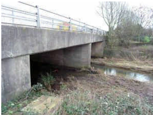
View of southern side of bridge looking east towards P&R site
