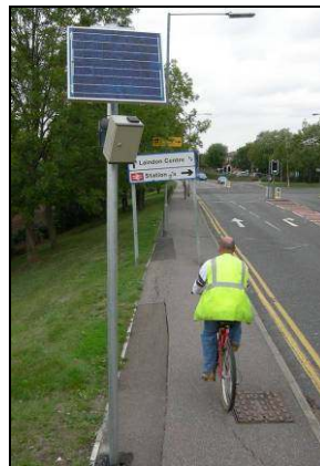
Solar panels at radar detector sites (detector and counting equipment in box below panel)
