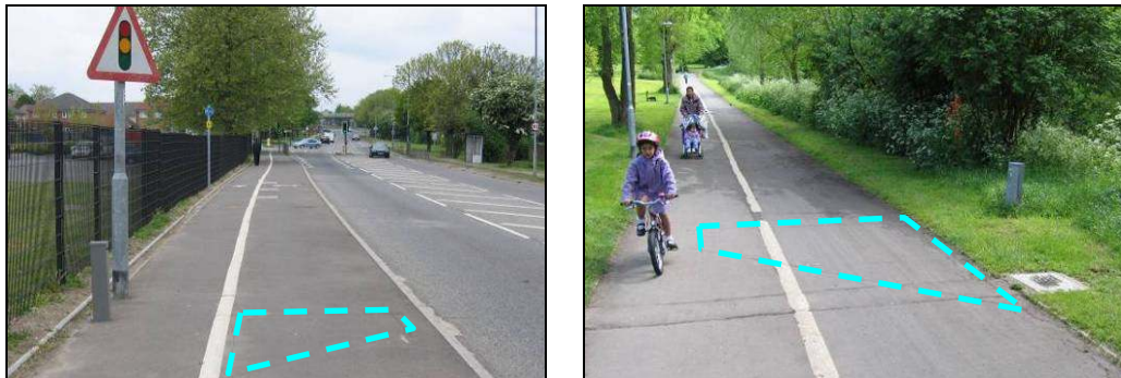
Inductive detection loops (highlighted) not covering full width of path
