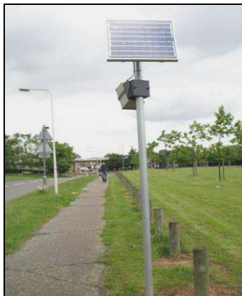
Solar panels at radar detector sites (detector and counting equipment in box below panel)
