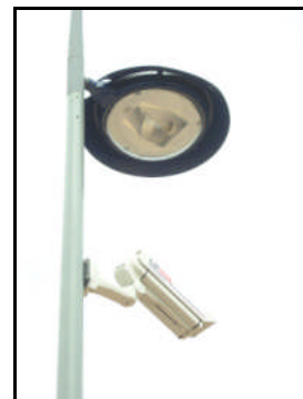
Lockers and CCTV at the Taunton park and ride site
