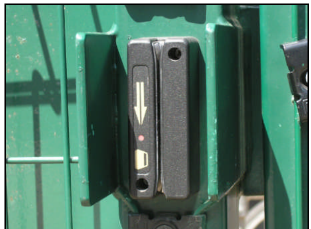
Close-up of swipe card lock Manchester University
