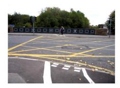
The arrangement above leads cyclists (and pedestrians) to this uncontrolled crossing of the A666. At no point do the signals stop traffic from all directions, while the expanse of carriageway to cross, and the inability to see the lights on the majority of signal heads from the vantage point of NMUs crossing, further adds to the challenge.
