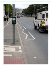
In locations, consideration has been given to cyclists both on and off the carriageway along parallel routes, so called 'dual provision'. This principle is to be endorsed, and applied more widely in the BwD area. That said, the on-road cycle lane in the picture is of sub-standard width and could be made wider without detriment to other road users.
