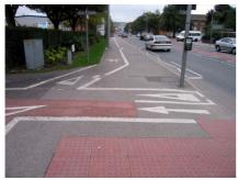
Here, the detailed layout (indicated by the surface markings) appears to cater for cyclists moving either parallel to the carriageway, or at right angles to this across the Toucan and into Blackburn College to the left of the picture. The arrangement does not readily lend itself to combining the two, at least if the surface markings are to be adhered to.
